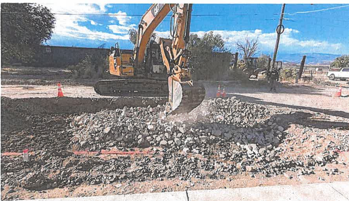
Placing 2 to 8-inch angular rock and applying pressure with trackhoe bucket
