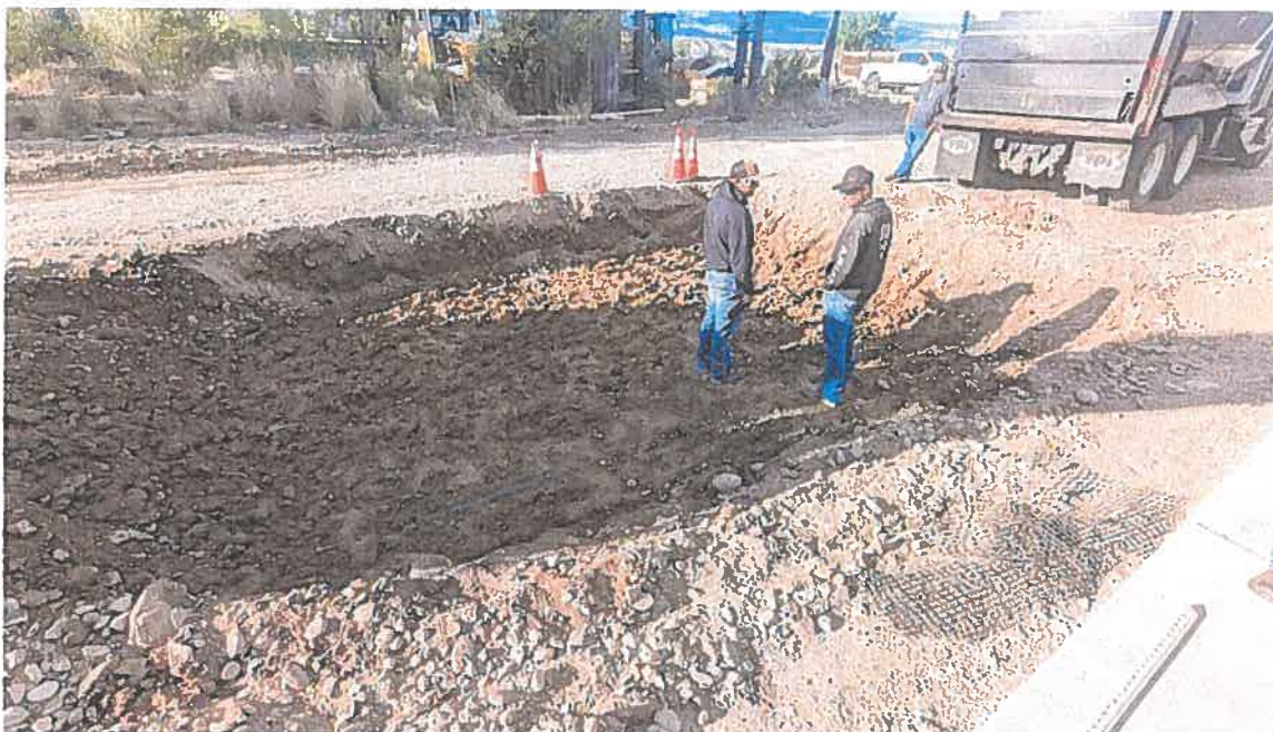
Bottom of subexcavated area within test section for revised stabilization approach
