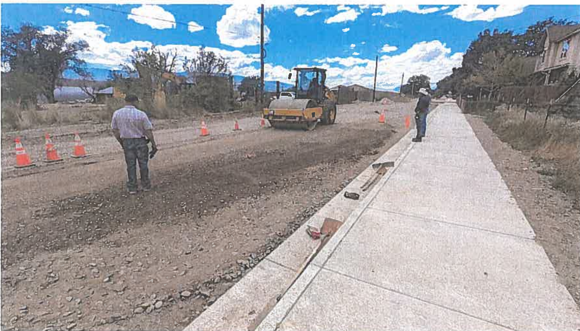
Compacting aggregate base course with steel-drum roller
