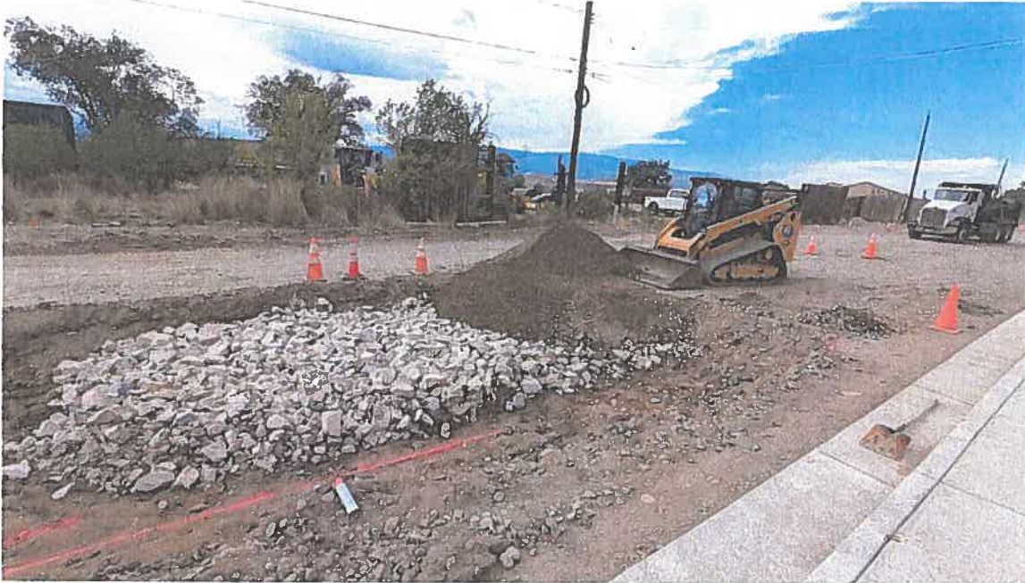
Placing 1.5-inch aggregate base course over the angular rock
